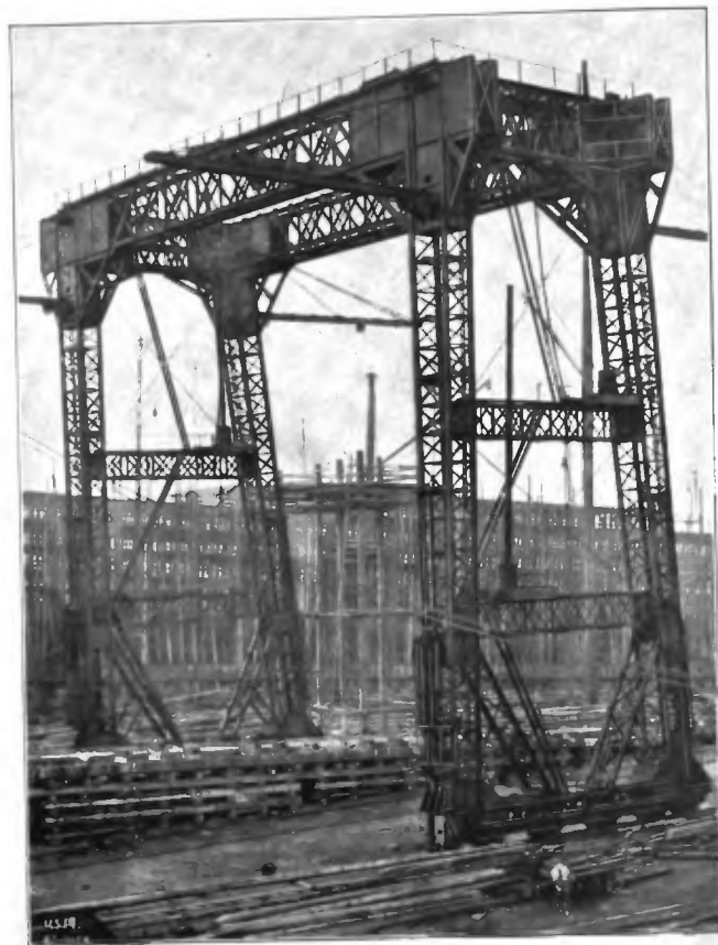
Fig. 81.—Gantry at Messrs Harland & Wolff's Shipbuilding Yard, Belfast.
